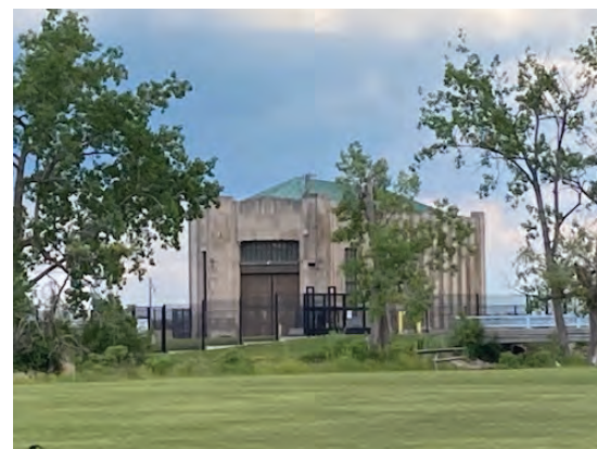
Intake Building on Belle Isle
