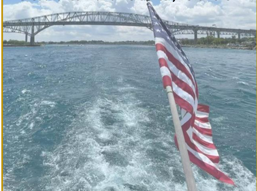
Blue Water Bridge
